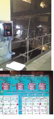
In the case of the Harris facility there is a switch located on the Rake gear drive. When the rake is at 90 degrees to the sensor the switch trips and sends the sensor down into the clarifier. In the case of this application we set the TSS sensor to trip at 3500 mg/l. The sensor will travel down into the clarifier and when it sees 3500 mg/l it will stop. The dept from the bottom of the clarifier is automatically indicated and outputted.
